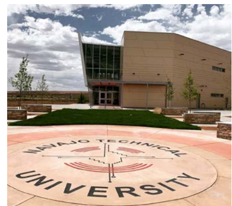
NTU's Chinle site's Academic Building finished construction in 2020.
